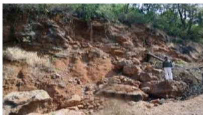
Fig. 12: Rockfall near Bhatgaon – (17°16’ N, 73° 24’ E).
